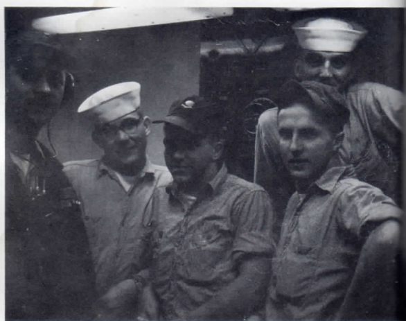
Pretty dark for the electrical shop.
