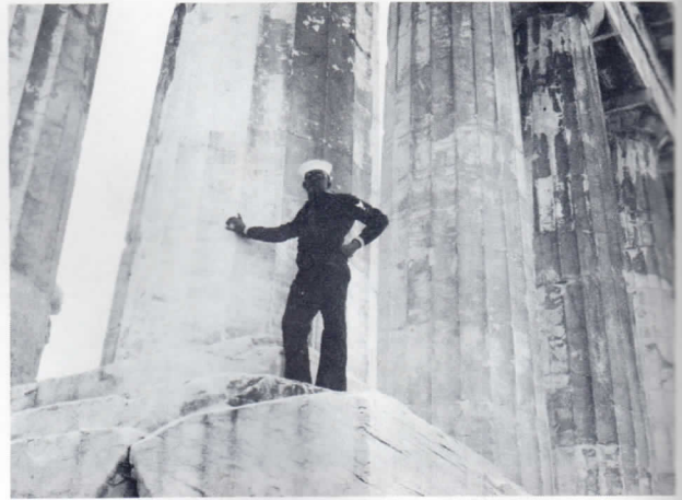
Needs a paint job.
